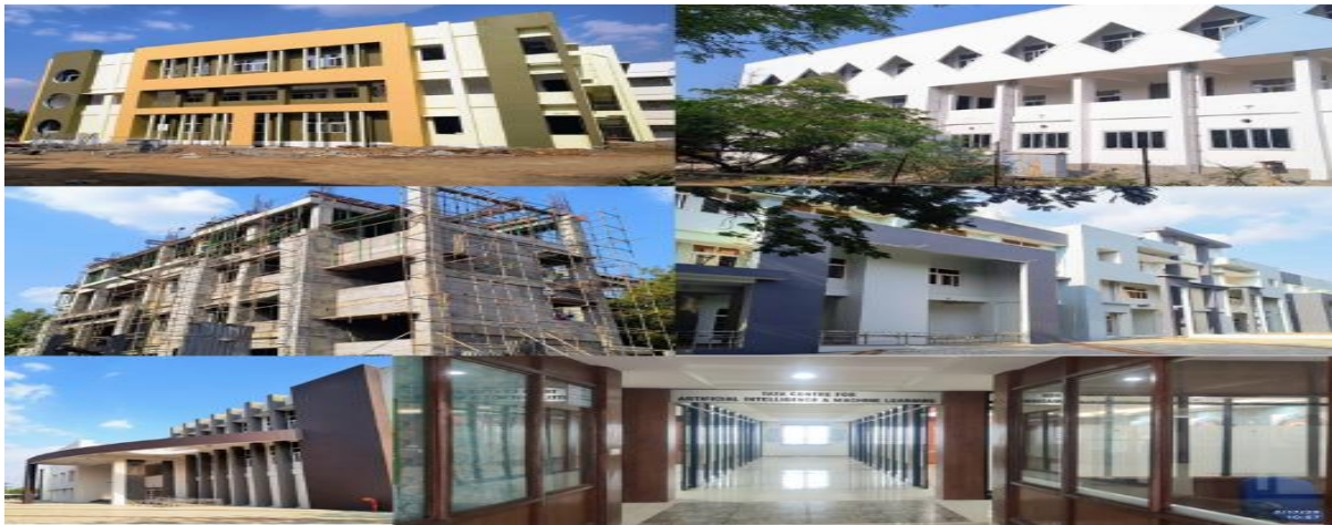
Six department's Annex buildings
