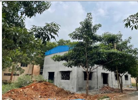
SCIEnT Expansion – Expansion of the facility through construction of Annex building
