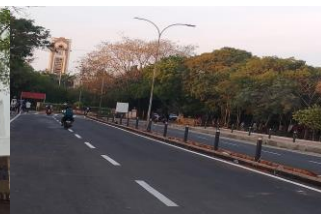
Road Widening and Recarpeting
