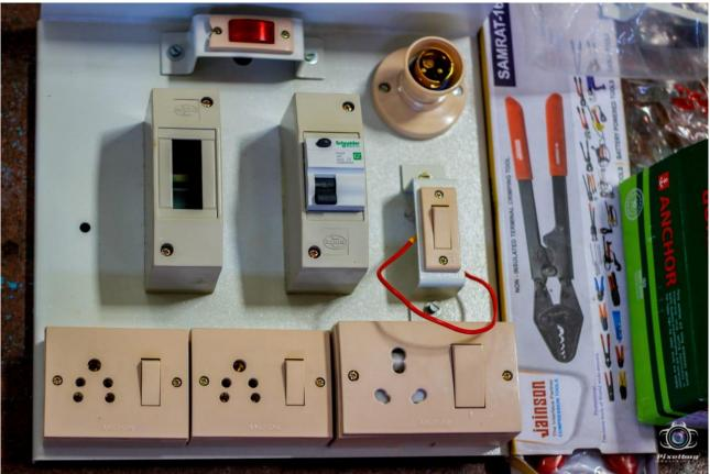
Photo: low-cost electric distribution board
